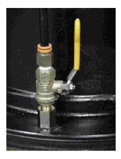
Note: Leave vent valve open in wet pit pump application to prevent air entrapment in jacket.
